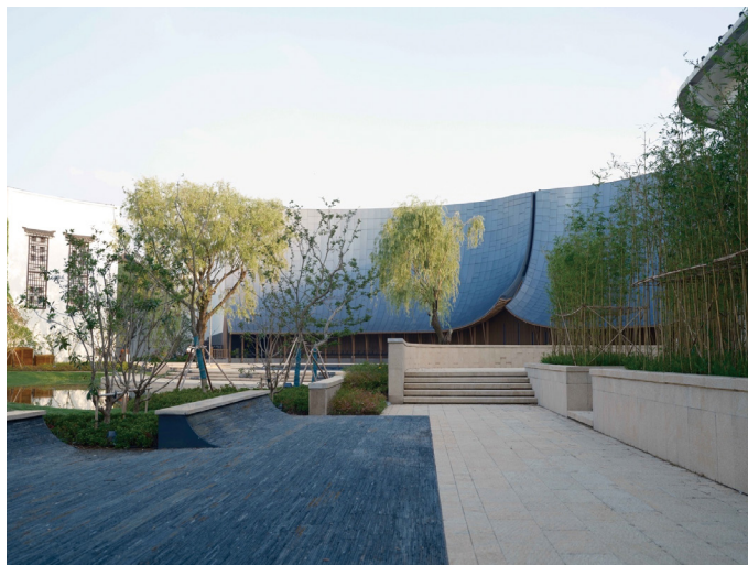
《只此周庄》演绎剧场改造 Zhouzhuang Theatre Renovation © 王赞 WANG Yun
